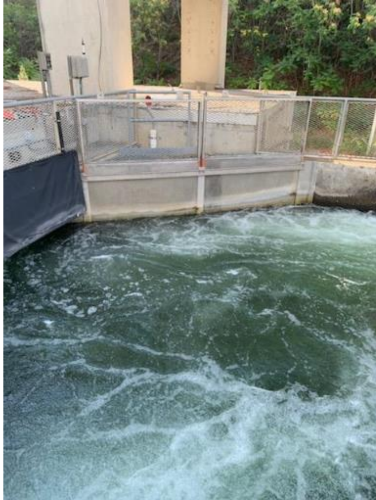
South ladder turning basin:
